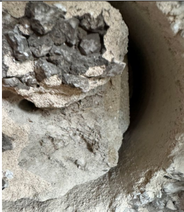
Figure 45: Alternative view to show pebble dash render finish with blockwork inner leaf.
