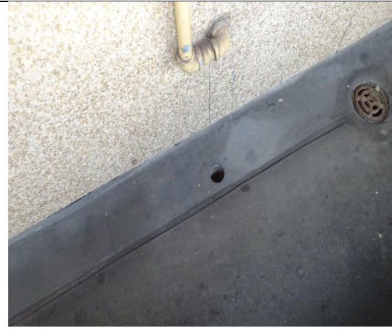
Figure 58: General view of redundant core holes through concrete floor slab to the open access balconies, which require fire stopping works to be completed.
