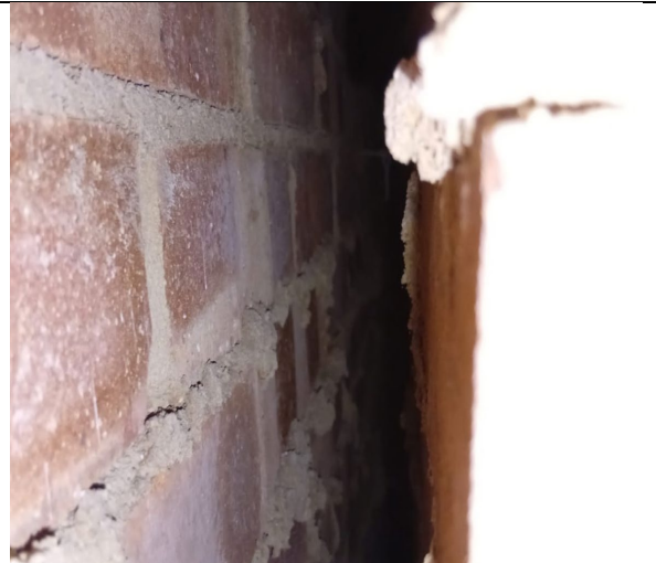
Figure 96: General view to show clear cavity.
