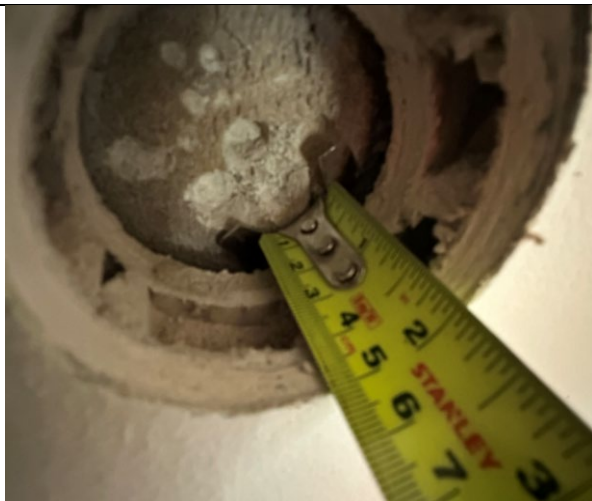
Figure 51: General view to show void between inner blockwork leaf and Paramount partition lining board – 10mm.
