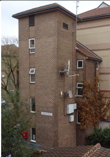
Figure 85: Alternative view of the traditional masonry cavity wall construction to the escape staircase located on the west elevation.
