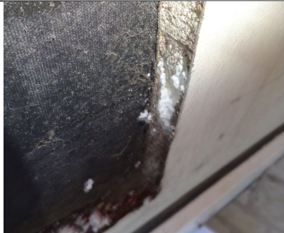
Figure 76: General view to show EPS insulated panel installed at low level to flat entrance door to Flat No. 354 (Harold Court).
