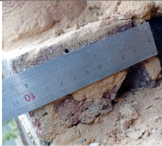
Figure 95: General view to confirm thickness outer brickwork leaf to window cill – 100mm.
