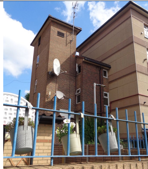
Figure 84: General view of the traditional masonry cavity wall construction to the escape staircase located on the west elevation.
