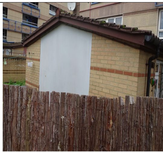
Figure 98: Alternative view of the traditional masonry cavity wall construction to the ground floor flats along the south elevation.
