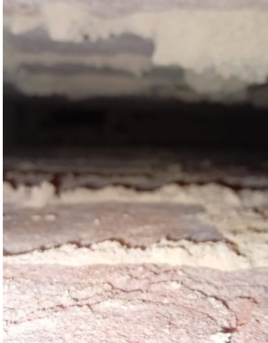
Figure 91: General view to show clear cavity below floor slab.
