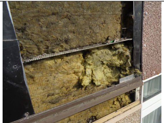
Figure 20: General view to show the Steni GRP rainscreen cladding panel and mineral wool insulation. NB. Some insulation is loose fixed and not mechanically fixed to concrete wall.
