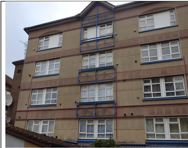
Figure 79: General view to show solid uPVC panels installed at fourth floor level along the south elevation.
