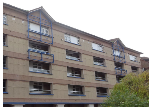
Figure 108: Alternative view of the architectural decorative steel attachments installed to the north elevation.
