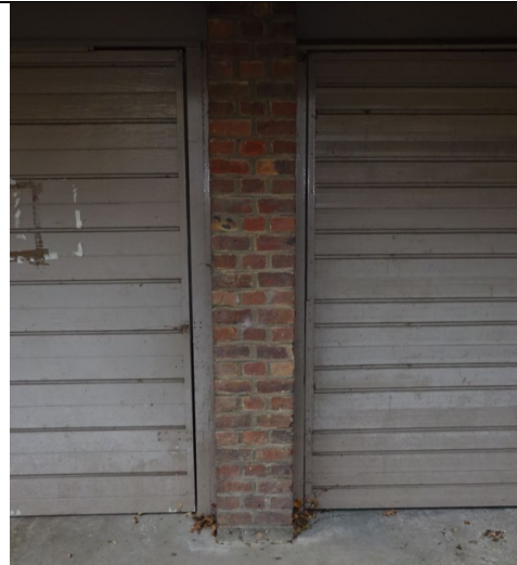
Figure 106: General view to show solid masonry wall located between garages.
