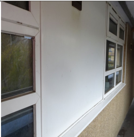
Figure 71: General view of the solid uPVC panels installed along the open access balconies located along the north elevation.
