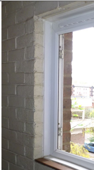
Figure 83: General view of the wall construction to show brick inner leaf and brick outer leaf.
