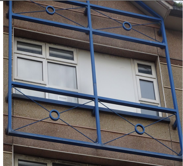
Figure 110: Alternative view of the decorative architectural steel attachments installed to the south elevation.
