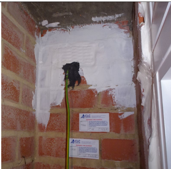
Figure 87: General view to show fire stopping works including ID labels completed to riser cupboards located in escape staircases (Albert Court).
