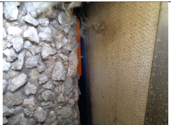
Figure 22: General view to missing insulation to window jamb.
