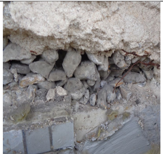
Figure 18: General view to show Wimpey no fines concrete.
