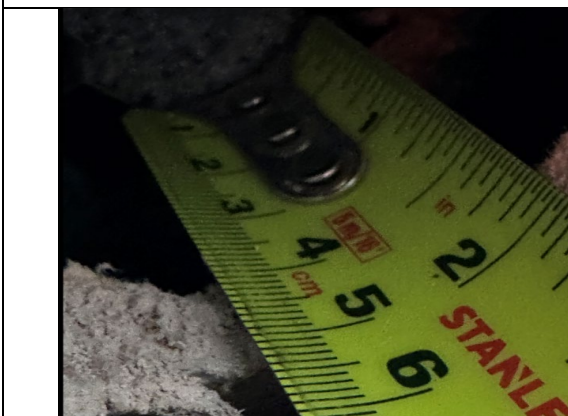
Figure 29: General view to show void between inner blockwork leaf and Paramount partition lining board – 40mm.
