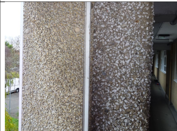
Figure 68: Close up view of Steni GRP rainscreen cladding panel installed over pebble dash render finish.
