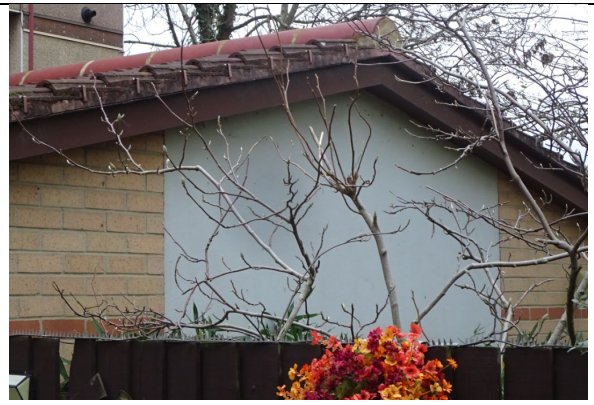
Figure 100: Alternative view of the traditional masonry cavity wall construction to the ground floor flats along the south elevation.
