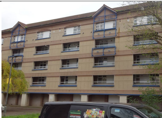
Figure 107: General view of the decorative architectural steel attachments installed to the north elevation.
