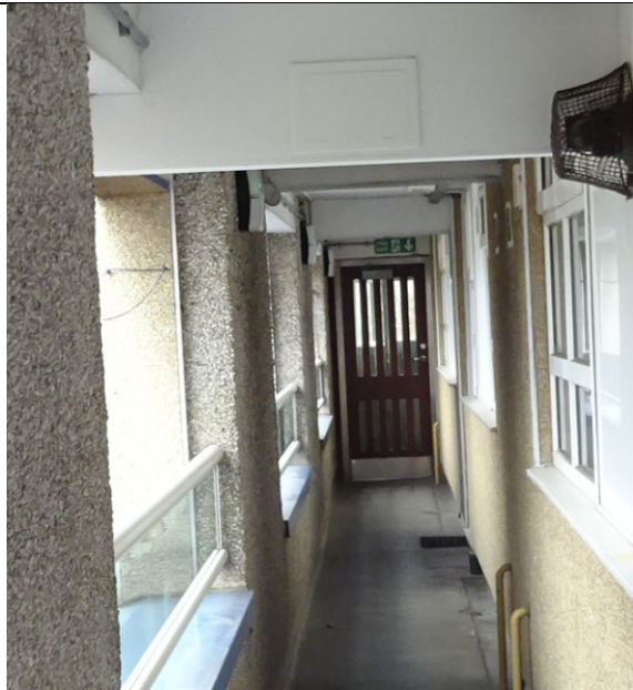
Figure 55: General view of Fire Door installed at the end of the open access balcony prior to entering the escape staircase.
