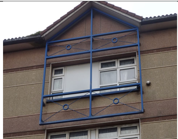
Figure 80: Close up view of the solid uPVC panels installed at fourth floor level along the south elevation.
