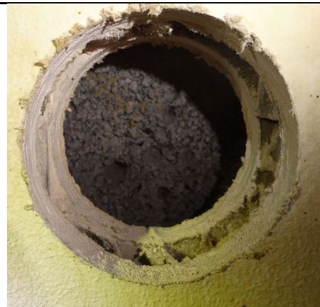
Figure 28: Close up view of the internal Paramount partition lining to the external wall.
