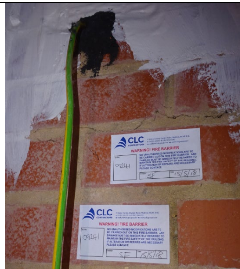
Figure 88: Close up view to show fire stopping works including ID labels completed to riser cupboards located in escape staircases (Albert Court).
