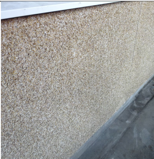
Figure 37: Close up view of the Steni GRP panels installed along the open access balconies.
