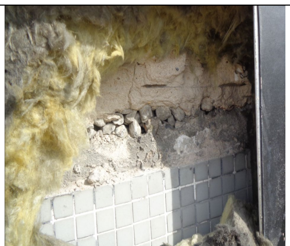
Figure 24: General view to show mineral wool insulation, pebble dash render with Wimpey no fines concrete.
