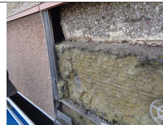
Figure 62: Alternative view of compartment floor detail, which shows mineral wool insulation installed at compartment floor location, but this does not fully fill the void behind the Steni GRP rainscreen cladding panel and the concrete floor slab (Taken from Queens Court 2021).
