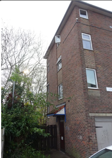
Figure 81: General view of the traditional masonry cavity wall construction to the escape staircase located on the east elevation.
