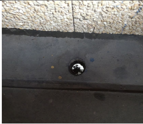
Figure 57: General view of redundant core holes through concrete floor slab to the open access balconies, which require fire stopping works to be completed.
