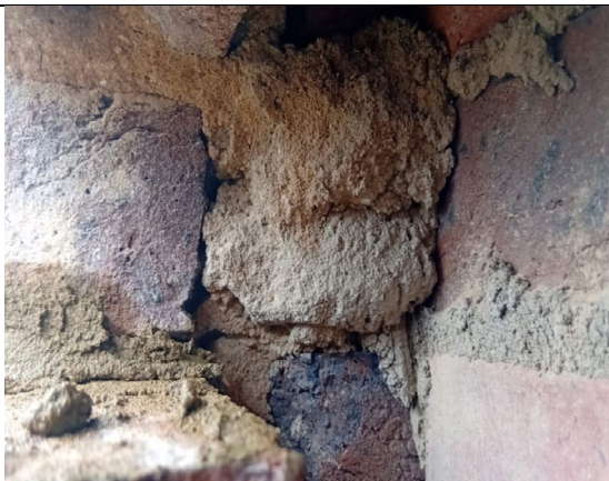
Figure 93: General view of window cill sample location to confirm that masonry wall closes the cavity.
