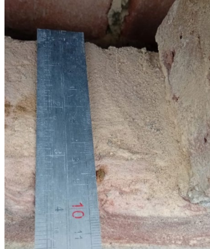
Figure 92: General view to confirm thickness of outer brickwork leaf – 100mm.
