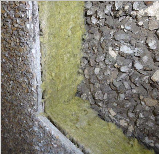
Figure 41: General view to show mineral wool insulation batt installed behind Steni GRP rainscreen cladding panel, with pebble dash render finish in the background.
