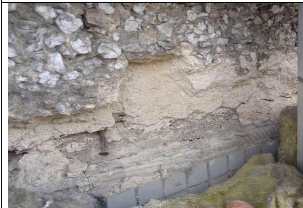
Figure 21: Close up view to show pebble dash render with Wimpey no fines concrete located behind render finish.
