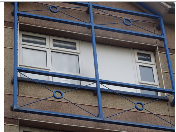
Figure 78: Close up view of the solid uPVC panels installed at fourth floor level along the north elevation.
