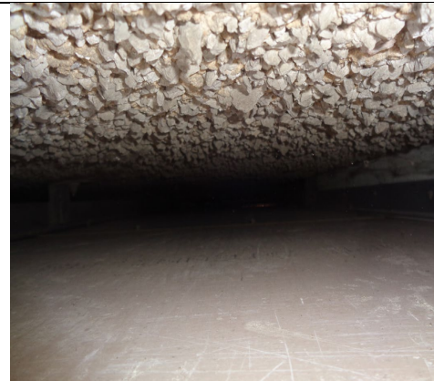
Figure 66: General view to show clear cavity between pebble dash render and the Steni GRP rainscreen cladding panel (Taken from Queens Court 2021).
