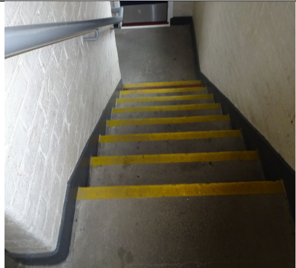
Figure 86: General view to show inner brick leaf and concrete escape staircase.
