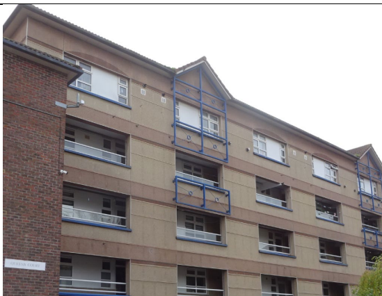
Figure 77: General view to show solid uPVC panels installed at fourth floor level along the north elevation.
