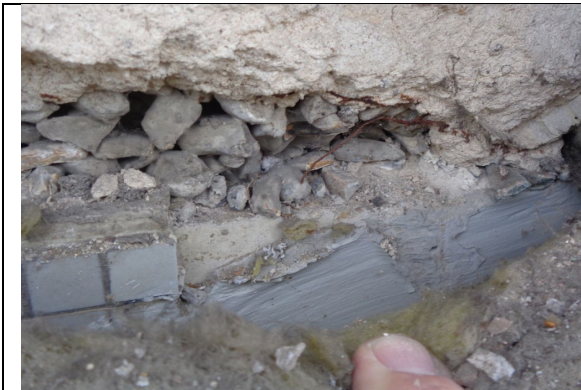
Figure 63: Close up view to show pebble dash render, Wimpey no fine concrete, concrete floor slab and mineral wool insulation installed at compartment floor location (Taken from Queens Court 2021).
