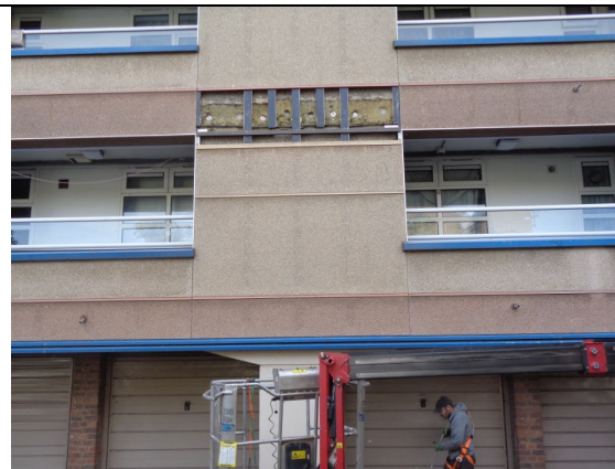
Figure 60: General view of compartment floor location to show no horizontal cavity barrier at compartment (Taken from Queens Court 2021).
