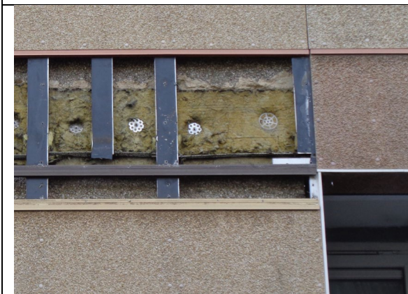
Figure 61: Close up view of compartment floor detail, which shows mineral wool insulation installed at compartment floor location, but this does not fully fill the void behind the Steni GRP rainscreen cladding panel (Taken from Queens Court 2021).
