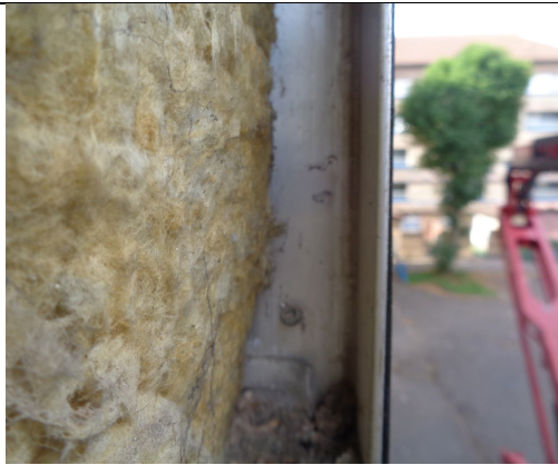
Figure 65: Close up view at compartment floor location to show that the mineral wool insulation does not fully fill the void and therefore does not form a suitable cavity barrier at compartment floor location (Taken from Queens Court 2021)
