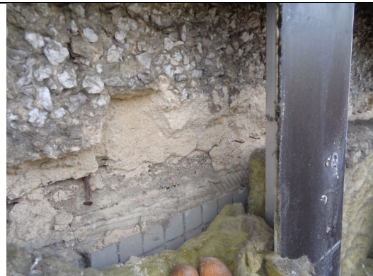
Figure 64: Alternative view to show pebble dash render, Wimpey no fine concrete, concrete floor slab and mineral wool insulation installed at compartment floor location (Taken from Queens Court 2021).
