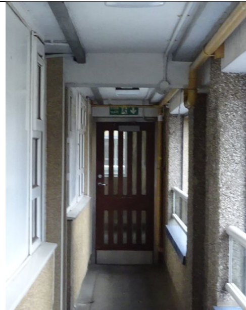
Figure 56: General view to show Fire Door installed at the opposite end of the open access balcony prior to entering the escape staircase and the concrete soffit to the open access balcony.
