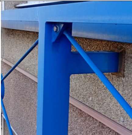
Figure 111: Close up view of the decorative architectural steel attachments installed (Albert Court).
