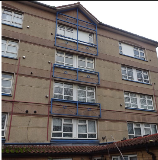
Figure 109: General view of the decorative architectural steel attachments installed to the south elevation.
