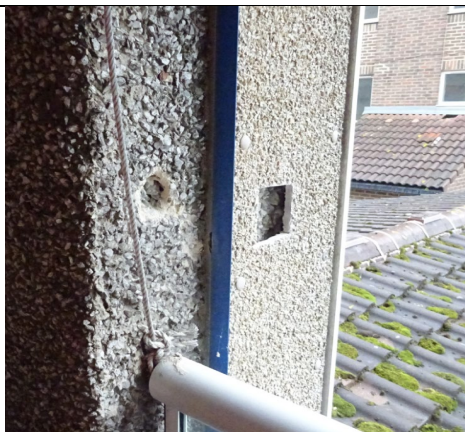
Figure 67: General view of sample locations to open access balcony wall reveals at first floor level (Harold Court).
