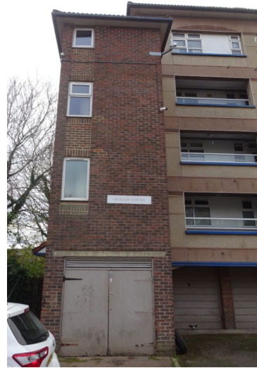
Figure 82: Alternative view of the traditional masonry cavity wall construction to the escape staircase located on the east elevation.
