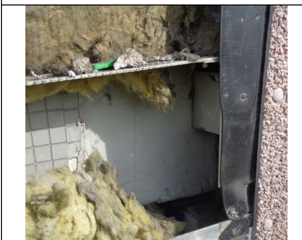
Figure 23: General view to show Steni GRP rainscreen cladding panel, stainless steel helping hand brackets and mineral wool insulation.
