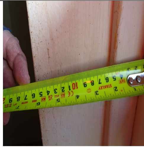
Figure 54: General view to confirm thickness of internal window reveal – 155mm.
