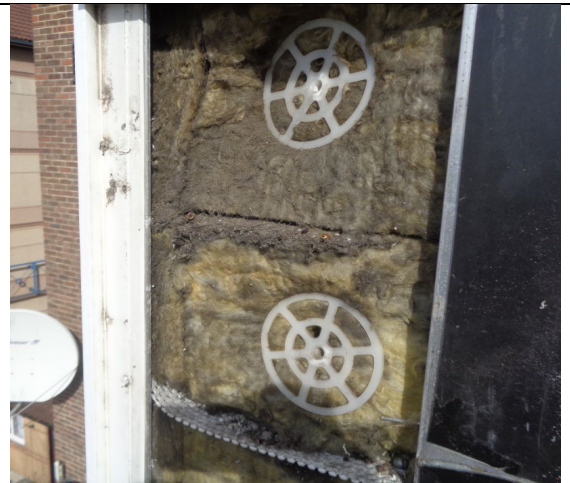
Figure 26: General view to show insulation mechanically fixed.
