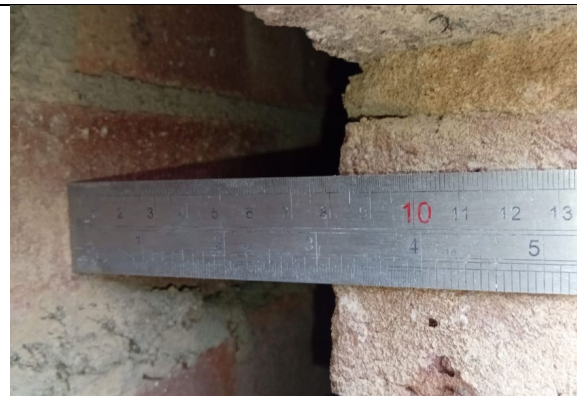
Figure 92: General view to confirm thickness of outer brickwork leaf – 100mm.
