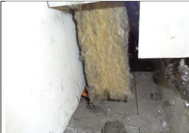
Figure 19: General view to show loose mineral wool insulation at compartment floor location to south elevation. NB. Unsuitable cavity barrier installed at compartment floor location.
