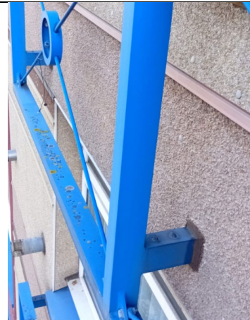
Figure 112: Close up view of the decorative architectural steel attachments installed (Albert Court).
