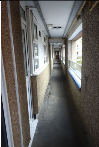
Figure 35: General view of the Steni GRP panels installed along the open access balconies along the north elevation at first floor level.
