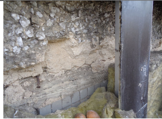
Figure 62: Alternative view to show pebble dash render, Wimpey no fine concrete, concrete floor slab and mineral wool insulation installed at compartment floor location (Taken from Queens Court 2021).
