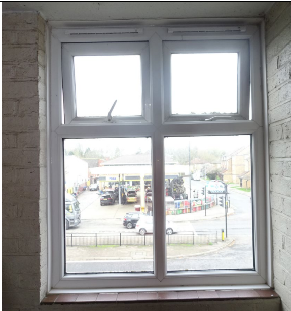
Figure 81: General view of the wall construction to show brick inner leaf.
