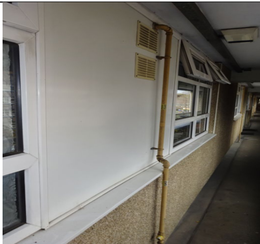
Figure 69: General view of the solid uPVC panels installed along the open access balconies located along the east elevation.
