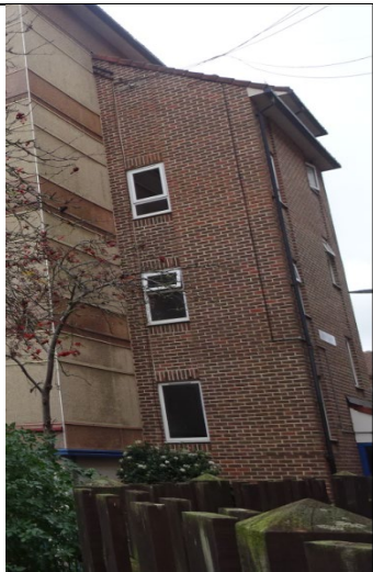
Figure 83: Alternative view of the traditional masonry cavity wall construction to the escape staircase located on the south elevation.
