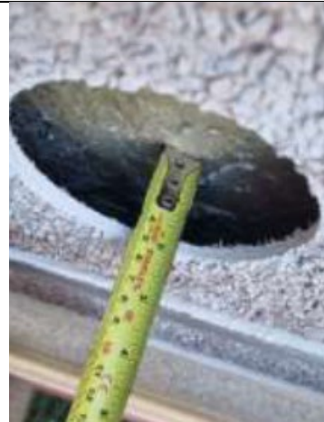
Figure 20: General view to show the Steni GRP rainscreen cladding panel and mineral wool insulation.
