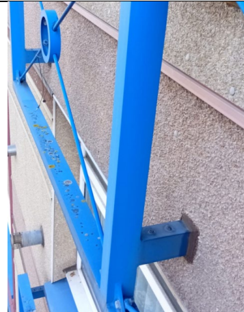
Figure 110: Close up view of the decorative architectural steel attachments installed.
