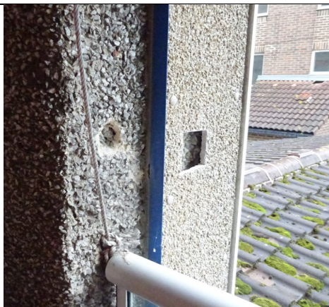
Figure 65: General view of sample locations to open access balcony wall reveals at first floor level (Taken from Harold Court).
