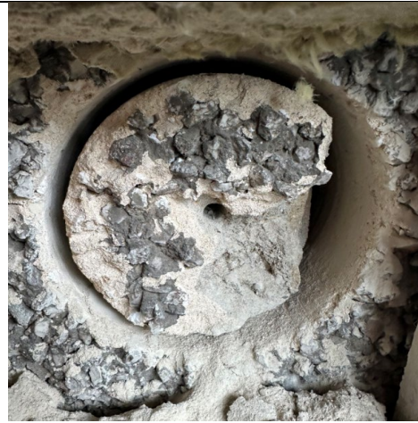
Figure 44: General view to show pebble dash render finish with blockwork inner leaf.
