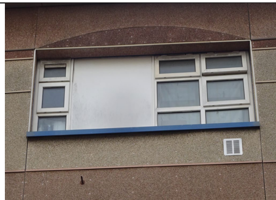
Figure 78: Close up view of the solid uPVC panels installed at fourth floor level along the west elevation.
