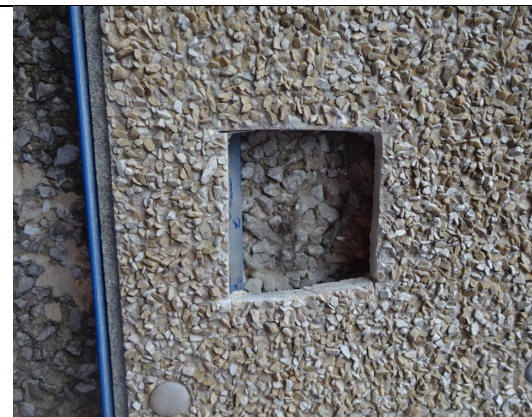
Figure 66: Close up view of Steni GRP rainscreen cladding panel installed over pebble dash render finish with 10mm void (Taken from Harold Court).
