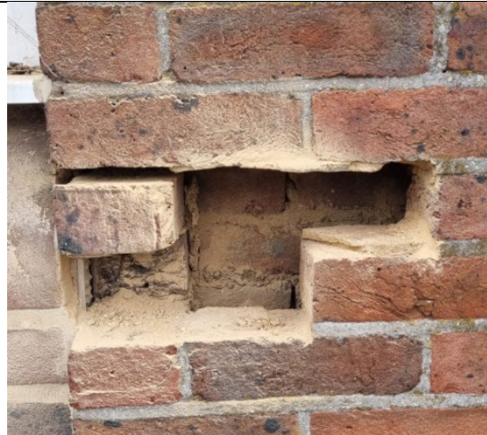
Figure 88: General view to show window cill cavity detail with masonry brickwork closing the cavity.
