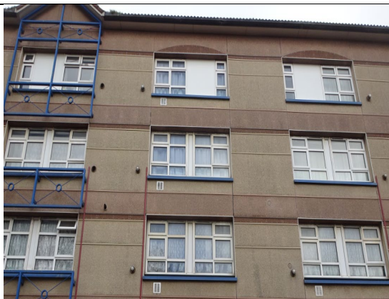
Figure 77: General view to show solid uPVC panels installed at fourth floor level along the west elevation.
