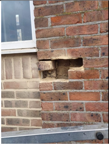
Figure 87: General view of sample location to window cill located on north elevation.
