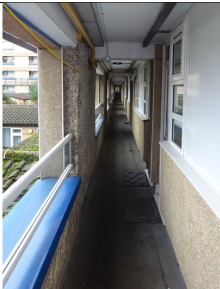
Figure 35: General view of the Steni GRP panels installed along the open access balconies along the east elevation at first floor level.
