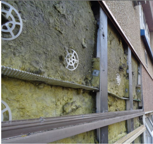
Figure 25: General view to show no horizontal cavity barrier installed at compartment floor location.
