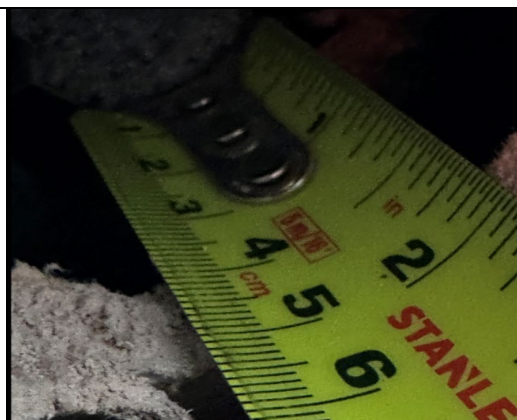
Figure 29: General view to show void between inner blockwork leaf and Paramount partition lining board – 40mm.
