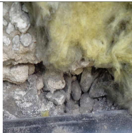
Figure 18: General view to show Wimpey no fines concrete.
