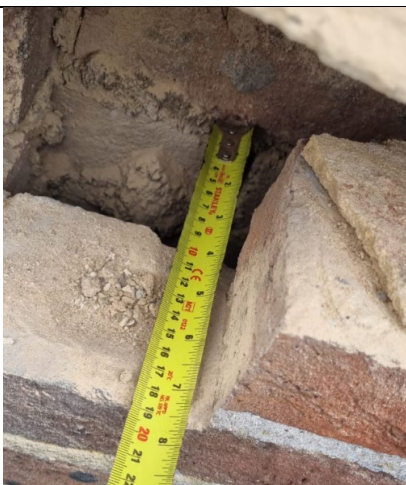
Figure 91: General view to confirm thickness of clear cavity – 90mm.
