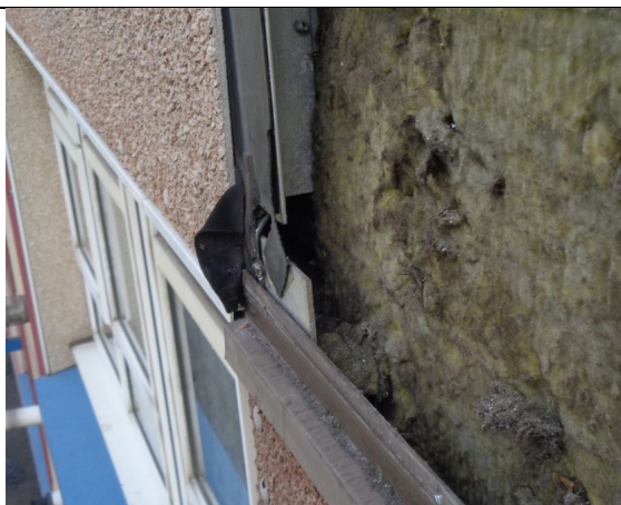
Figure 23: General view to show Steni GRP rainscreen cladding panel, stainless steel helping hand brackets and mineral wool insulation.
