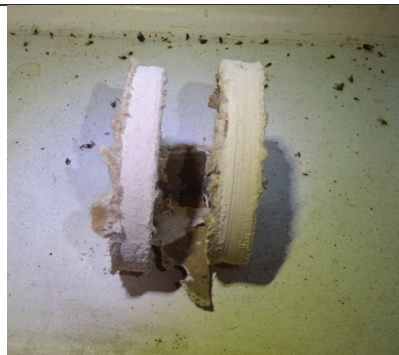
Figure 52: Close up view of Paramount partition lining board which comprises of two layers of 10mm plasterboard with an 18mm honeycomb cardboard core.
