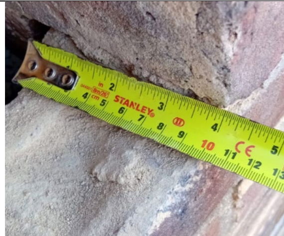
Figure 90: General view to confirm thickness of outer brickwork leaf – 100mm.
