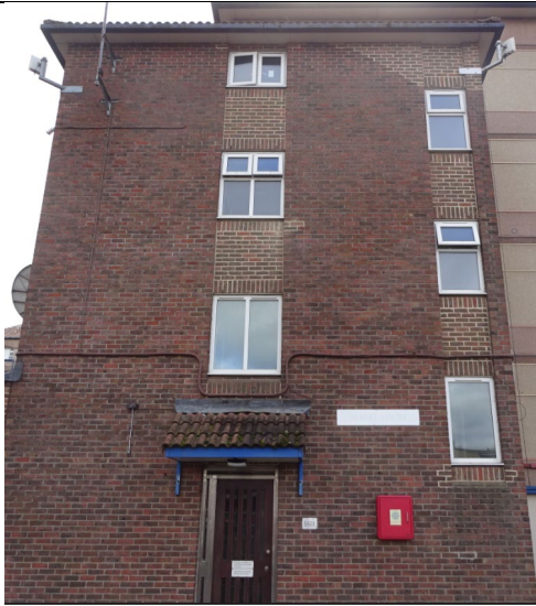
Figure 79: General view of the traditional masonry cavity wall construction to the escape staircase located on the north elevation.
