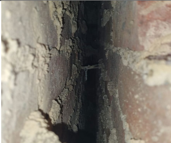
Figure 89: General view to show clear cavity.
