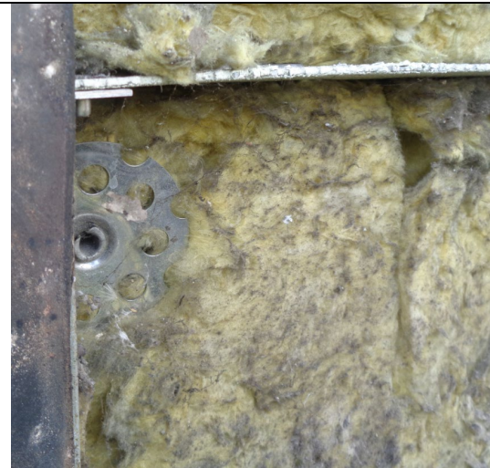
Figure 16: Close up view to show mineral wool insulation.
