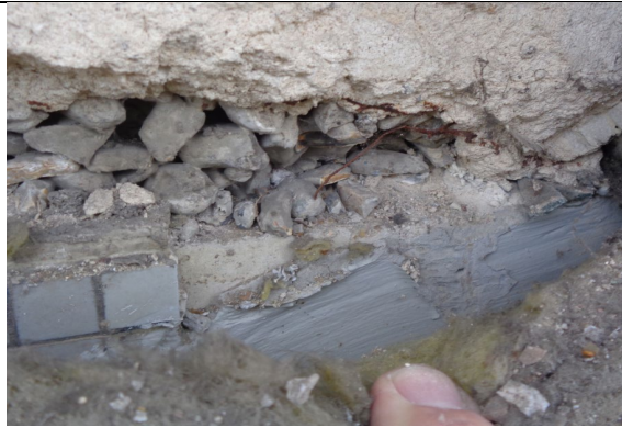
Figure 61: Close up view to show pebble dash render, Wimpey no fine concrete, concrete floor slab and mineral wool insulation installed at compartment floor location (Taken from Queens Court 2021).
