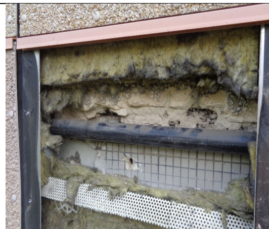
Figure 24: General view to show service pipes / cables located with mineral wool insulation.
