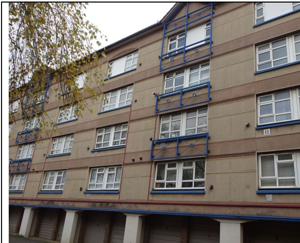
Figure 105: General view of the decorative architectural steel attachments installed to the west elevation.
