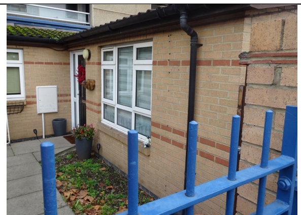
Figure 96: Alternative view of the traditional masonry cavity wall construction to the ground floor flats along the east elevation.
