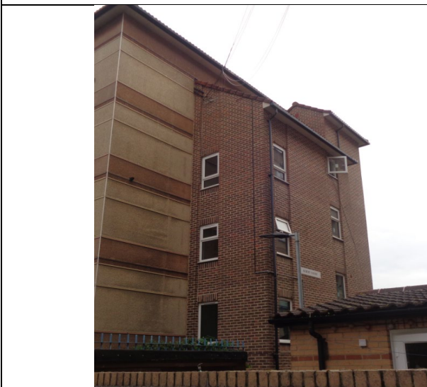
Figure 3: Rear (South) elevation of the building.
