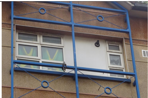
Figure 76: Close up view of the solid uPVC panels installed at fourth floor level along the east elevation.
