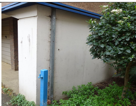
Figure 103: General view of the reinforced concrete wall to the south elevation at ground floor level.
