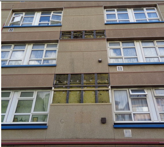
Figure 15: General view of External Wall Type #1.
