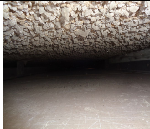
Figure 64: General view to show clear cavity between pebble dash render and the Steni GRP rainscreen cladding panel (Taken from Queens Court 2021).
