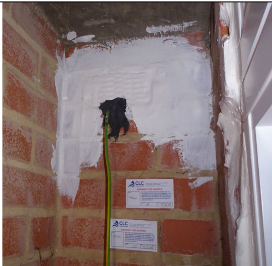
Figure 85: General view to show fire stopping works including ID labels completed to riser cupboards located in escape staircases.
