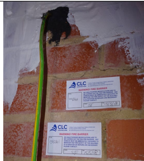
Figure 86: Close up view to show fire stopping works including ID labels completed to riser cupboards located in escape staircases.
