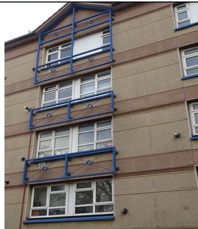
Figure 106: Alternative view of the architectural decorative steel attachments installed to the west elevation.
