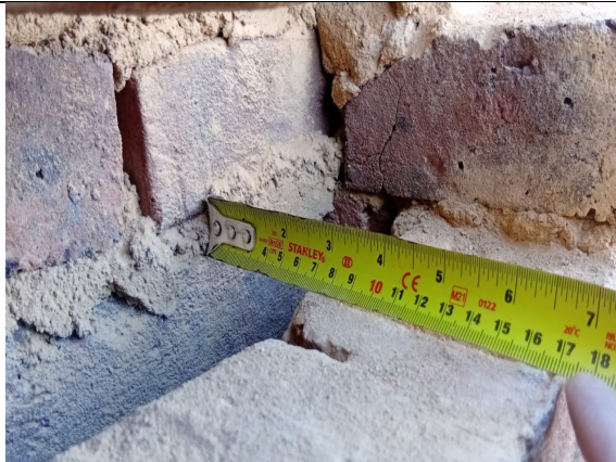
Figure 93: General view to confirm thickness of cavity -70mm and outer brickwork leaf - 100mm at compartment floor location.
