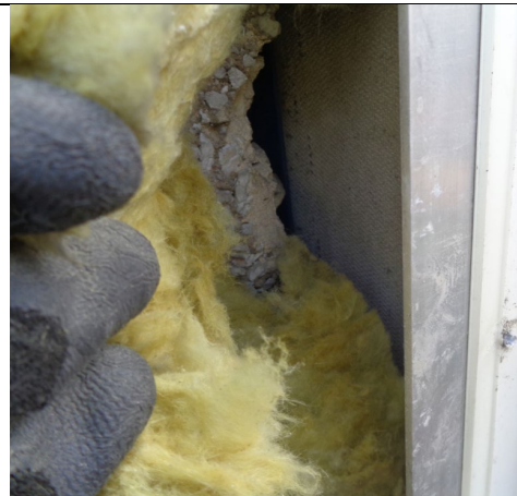
Figure 22: General view to missing insulation to window jamb.
