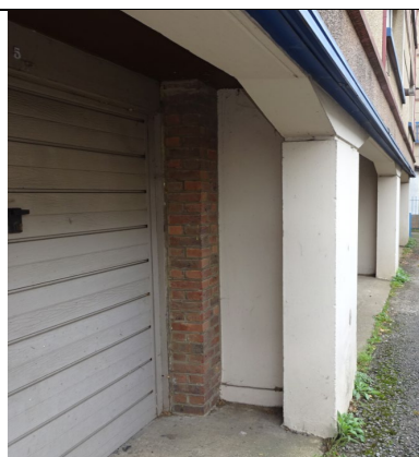
Figure 102: Close up view to show reinforced concrete wall and frame to the west elevation.
