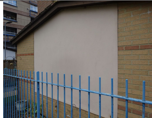
Figure 98: Alternative view of the traditional masonry cavity wall construction to the ground floor flats along the east elevation.
