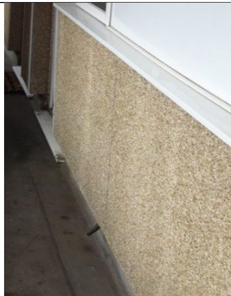
Figure 36: Close up view of the Steni GRP panels installed along the open access balconies.
