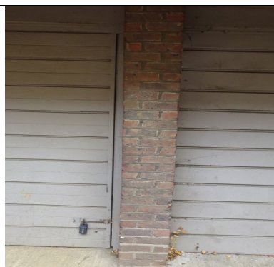
Figure 104: General view to show solid masonry wall located between garages.
