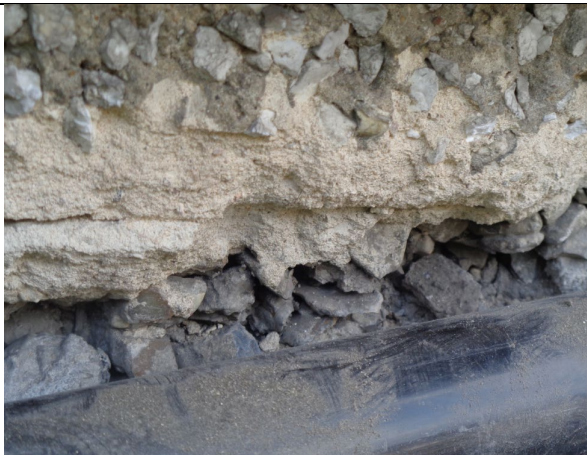
Figure 21: Close up view to show pebble dash render with Wimpey no fines concrete located behind render finish.
