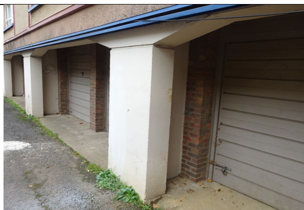
Figure 101: General view of the reinforced concrete frame and concrete floor to the west elevation. NB. that the garages are recessed back from the main elevation.
