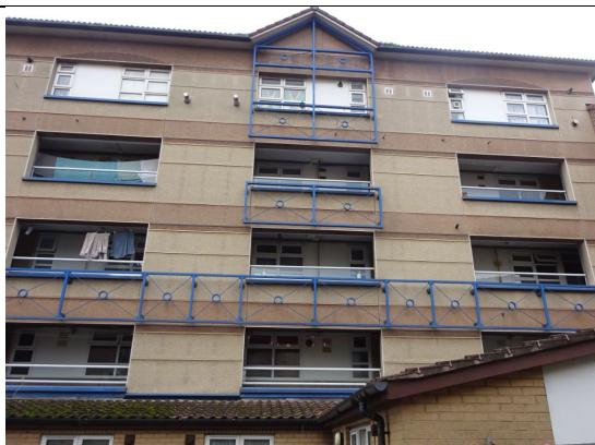
Figure 75: General view to show solid uPVC panels installed at fourth floor level along the east elevation.
