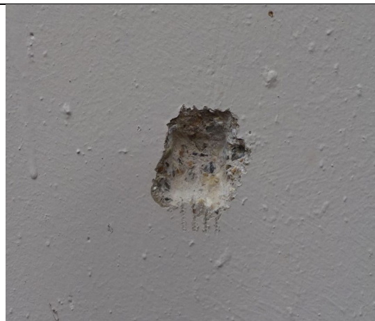
Figure 100: Close up view of the sample location to confirm solid concrete shear wall (Harold Court).
