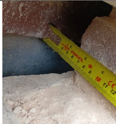
Figure 94: General view to show concrete floor slab, 160mm deep and confirm cavity thickness - 70mm.
