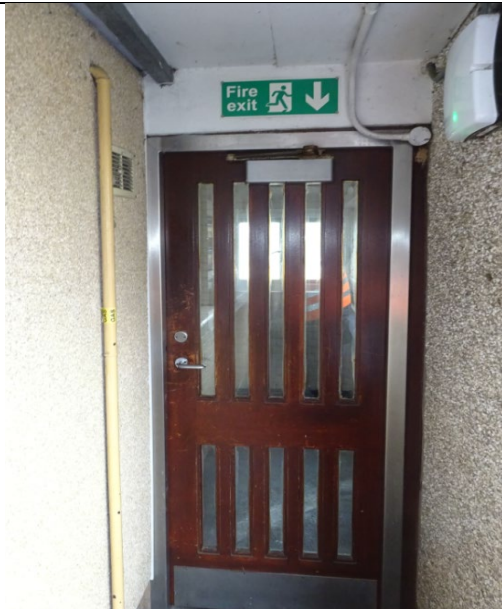
Figure 55: General view of Fire Door installed at the end of the open access balcony prior to entering the escape staircase.
