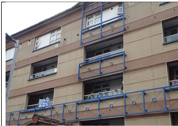
Figure 57: General view of External Wall Type #3
