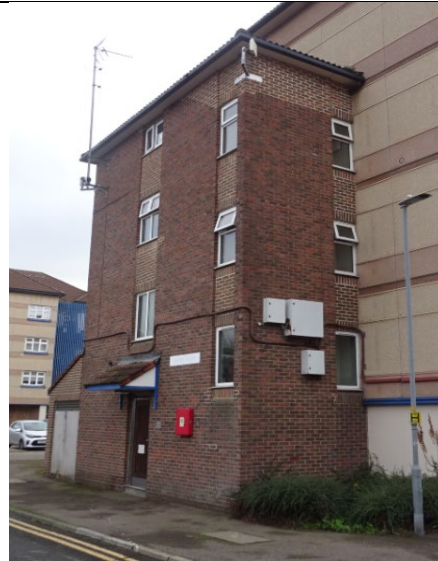
Figure 80: Alternative view of the traditional masonry cavity wall construction to the escape staircase located on the north elevation.
