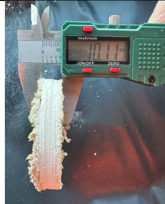
Figure 34: General view to confirm thickness of the plasterboard – 10mm.
