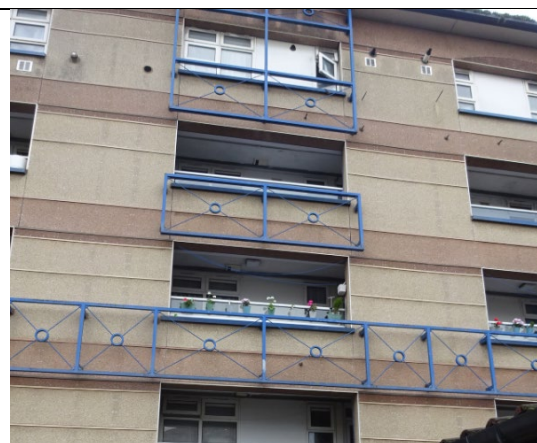
Figure 108: Alternative view of the decorative architectural steel attachments installed to the east elevation.
