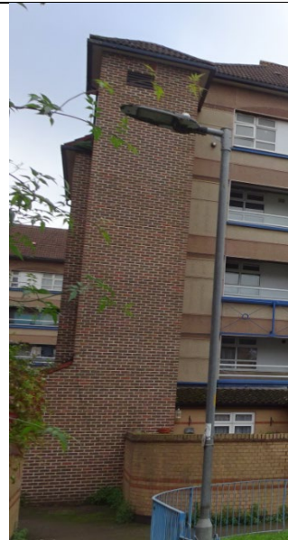
Figure 82: General view of the traditional masonry cavity wall construction to the escape staircase located on the south elevation.
