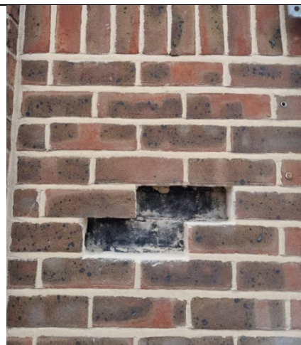
Figure 92: General view of sample location at compartment floor location to north elevation.
