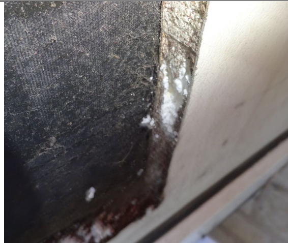
Figure 74: General view to show EPS insulated panel installed at low level to flat entrance door to Flat No. 354 (Harold Court).
