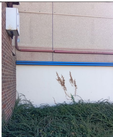
Figure 99: General view of the reinforced concrete wall to the north elevation at ground floor level, showing sample location.
