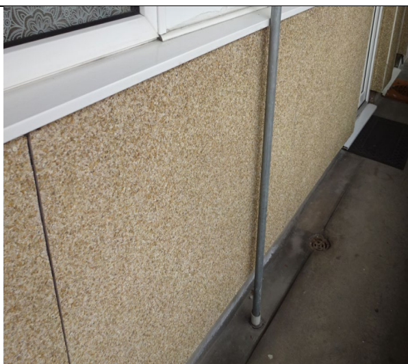
Figure 37: Close up view of the Steni GRP panels installed along the open access balconies.
