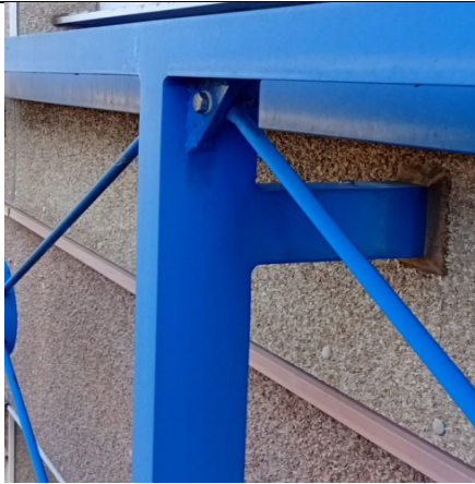
Figure 109: Close up view of the decorative architectural steel attachments installed.
