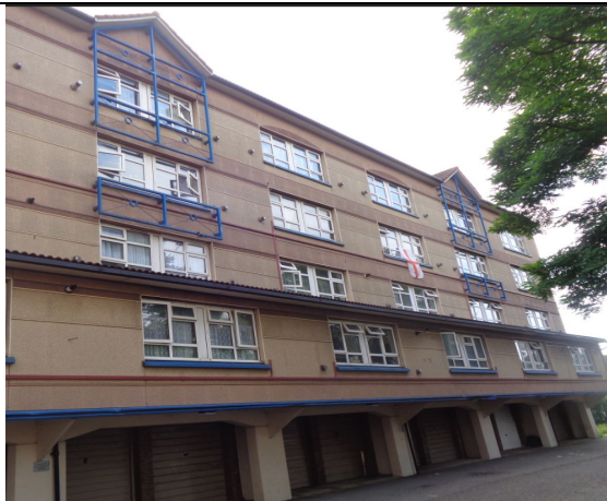
Figure 121: General view of the decorative architectural steel attachments installed to the west elevation.
