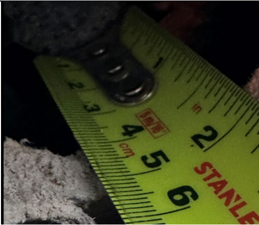
Figure 47: General view to show void between inner blockwork leaf and Paramount partition lining board – 40mm.
