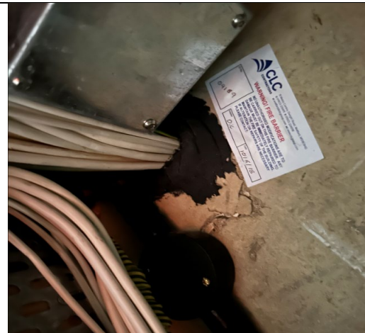
Figure 102: General view to show fire stopping works including ID labels completed to riser cupboards located in escape staircases (Harold Court).
