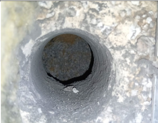
Figure 43: Alternative view to show 20mm pebble dash render, 60mm blockwork outer leaf, 50mm clear cavity and blockwork inner leaf.
