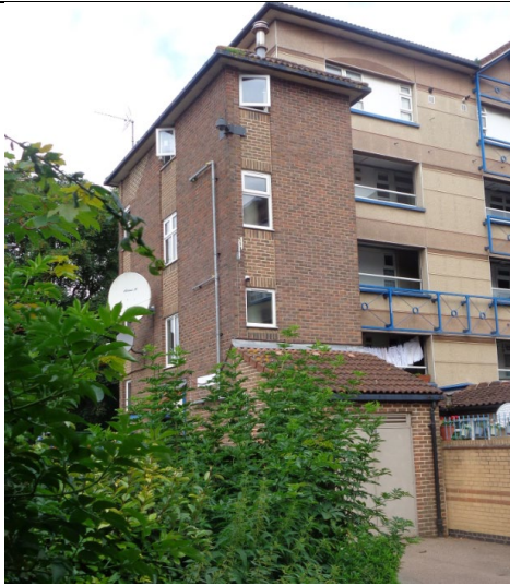
Figure 99: Alternative view of the traditional masonry cavity wall construction to the escape staircase located on the south elevation.
