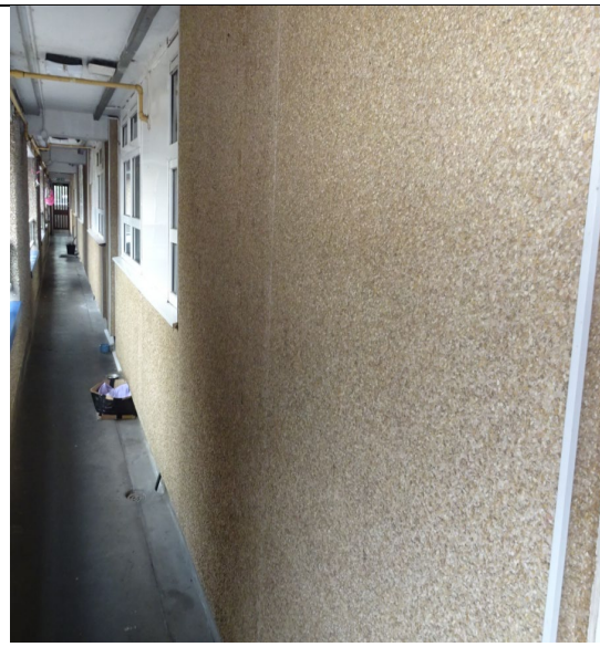
Figure 54: Close up view of the Steni GRP panels installed along the open access balconies.
