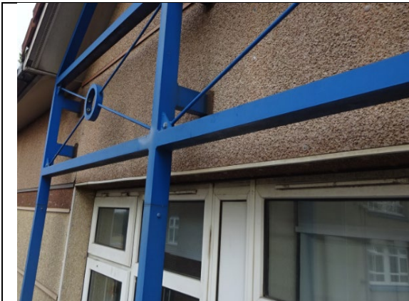
Figure 125: Close up view of the decorative architectural steel attachments installed to the west elevation.
