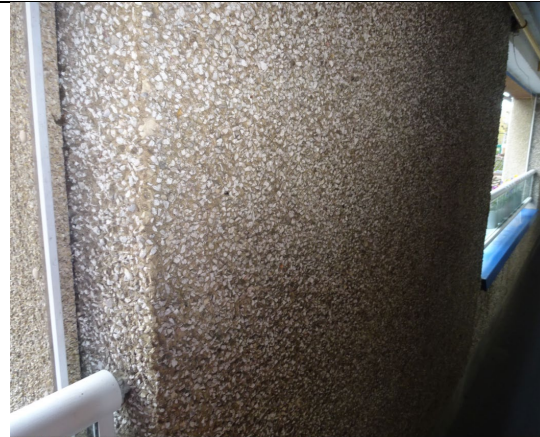
Figure 86 General view of pebble dash render finish to external wall of first floor open access balcony along the east elevation.
