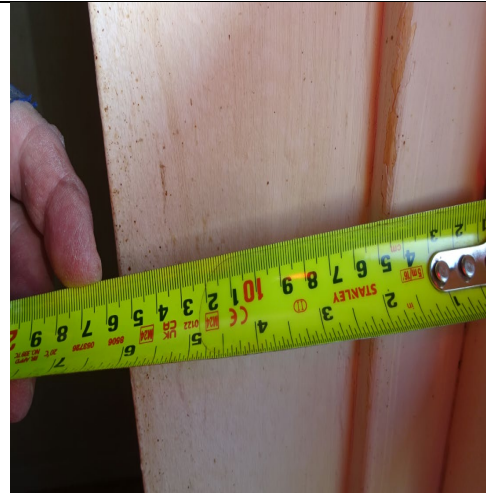
Figure 72: General view to confirm thickness of internal window reveal – 155mm.
