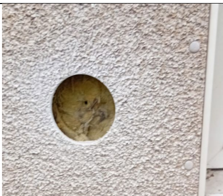
Figure 39: General view of sample location to show Steni GRP rainscreen cladding panel, cavity void and mineral wool insulation.
