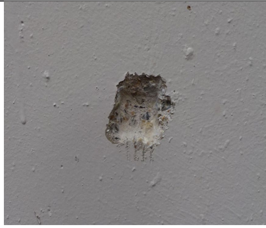
Figure 116: Close up view of the sample location to confirm solid concrete shear wall (Harold Court).
