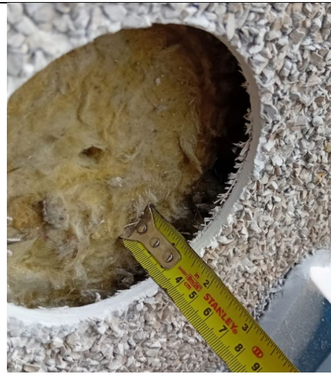
Figure 20: General view to show the Steni GRP rainscreen cladding panel, mineral wool insulation and Wimpey no fines concrete.
