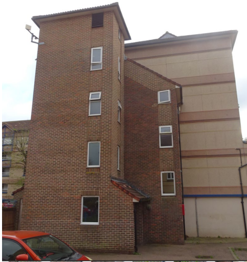
Figure 95: General view of the traditional masonry cavity wall construction to the escape staircase located on the north elevation.
