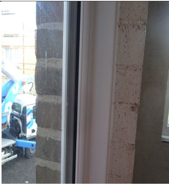
Figure 97: General view of the wall construction to show brick inner leaf and brick outer leaf.
