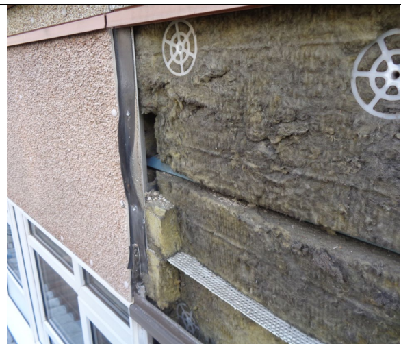
Figure 16: Close up view to show mineral wool insulation with limited mechanical fixings.
