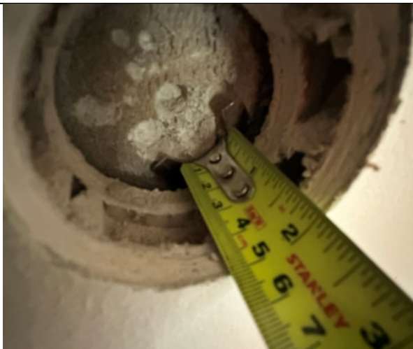
Figure 69: General view to show void between inner blockwork leaf and Paramount partition lining board – 10mm.
