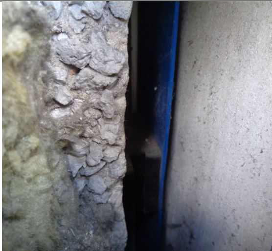
Figure 23: Alternative view to show no insulation installed to window jamb.
