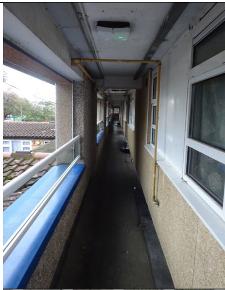
Figure 53: General view of the Steni GRP panels installed along the open access balconies along the east elevation at first floor level.
