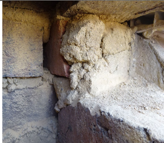
Figure 104: General view to show window cill cavity detail with masonry brickwork closing the cavity.
