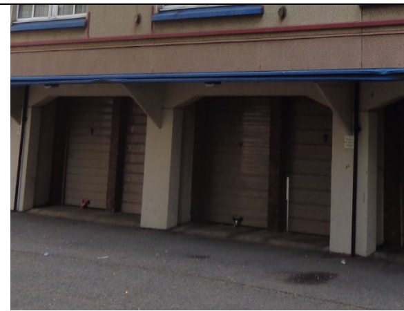
Figure 117: General view of the reinforced concrete frame and concrete floor to the west elevation. NB. that the garages are recessed back from the main elevation.
