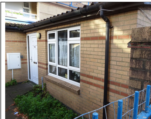
Figure 111: General view of the traditional masonry cavity wall construction to the ground floor flats along the east elevation.
