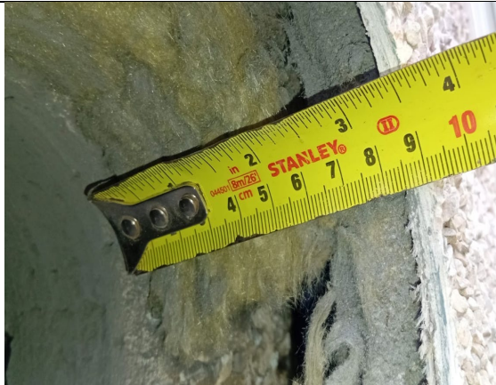
Figure 41: General view to show Steni GRP rainscreen cladding panel, mineral wool insulation pebble dash render and blockwork outer leaf.
