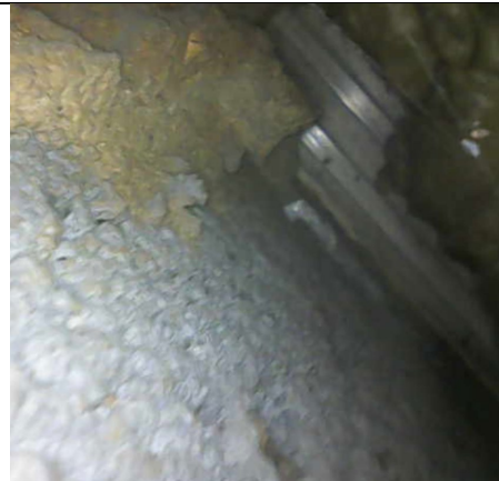
Figure 44: General view of clear cavity to blockwork outer and inner leaves to show uPVC cavity closer to window jamb (Harold Court).
