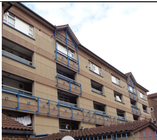
Figure 123: General view of the decorative architectural steel attachments installed to the east elevation.
