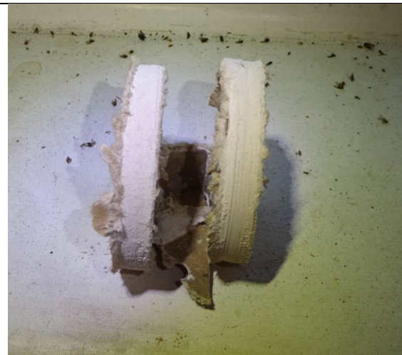
Figure 70: Close up view of Paramount partition lining board which comprises of two layers of 10mm plasterboard with an 18mm honeycomb cardboard core.
