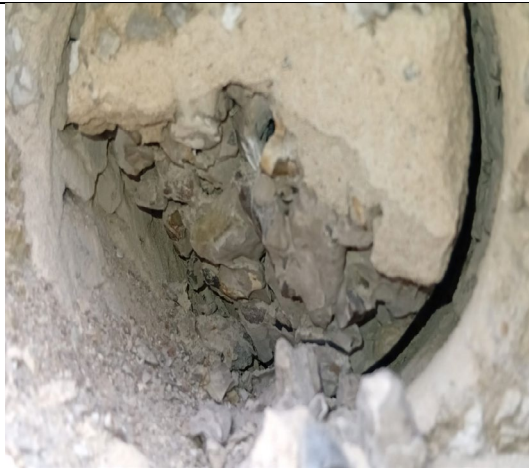
Figure 21: Close up view to show pebble dash render with Wimpey no fines concrete located behind render finish.
