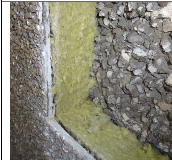
Figure 59: General view to show mineral wool insulation batt installed behind Steni GRP rainscreen cladding panel, with pebble dash render finish in the background.
