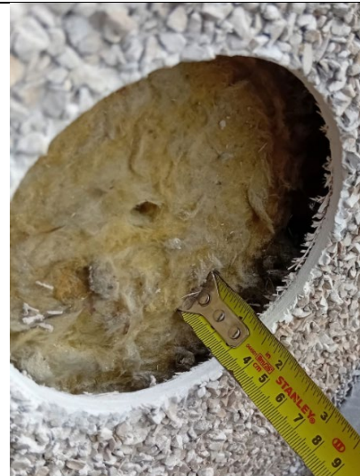
Figure 32: General view to show Steni GRP rainscreen cladding panel, cavity void and mineral wool insulation.
