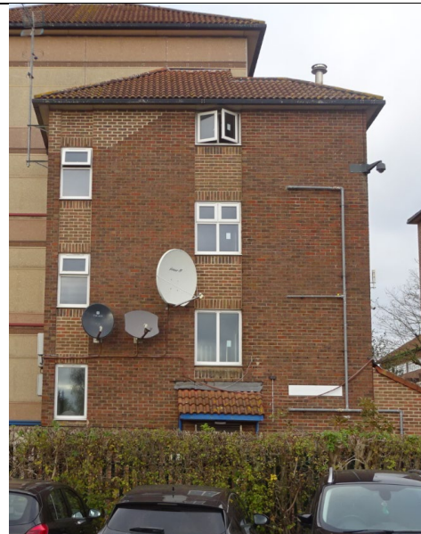
Figure 98: General view of the traditional masonry cavity wall construction to the escape staircase located on the south elevation.
