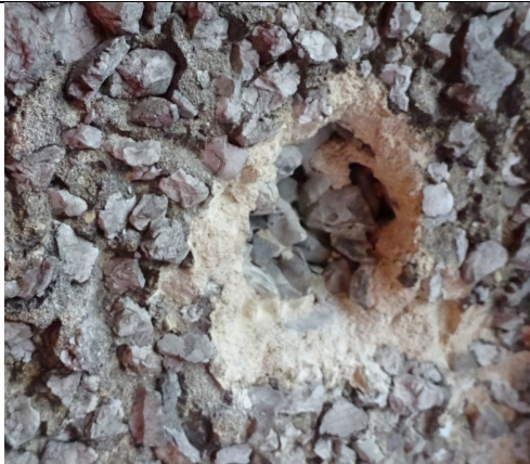
Figure 85 Close up view to show pebble dash render finish installed over Wimpey no fines concrete (Harold Court).
