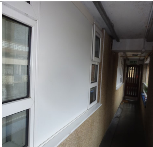
Figure 87: General view of the solid uPVC panels installed along the open access balconies located along the east elevation.
