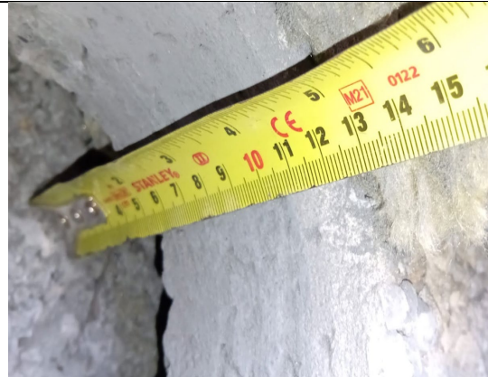
Figure 42: General view to show 60mm blockwork outer leaf, 50mm clear cavity and blockwork inner leaf.
