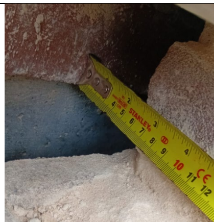
Figure 108: General view to confirm thickness of clear cavity between inner brickwork leaf and outer brickwork leaf – 60mm.
