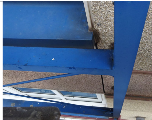
Figure 126: Close up view of the decorative architectural steel attachments installed to the west elevation.
