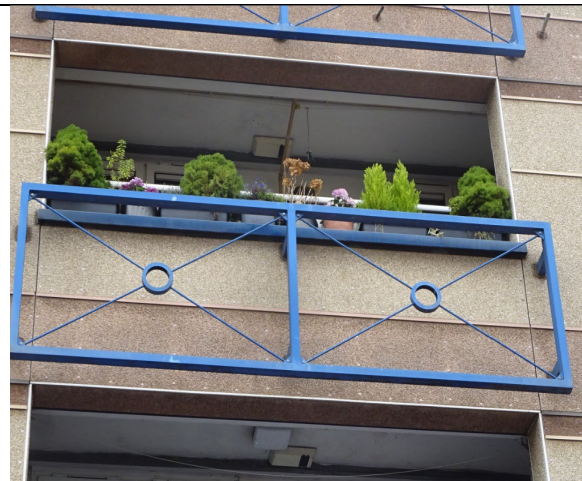
Figure 124: Alternative view of the decorative architectural steel attachments installed to the east elevation.
