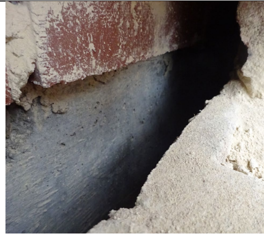
Figure 110: General view to show concrete slab to escape staircases – 160mm deep concrete.
