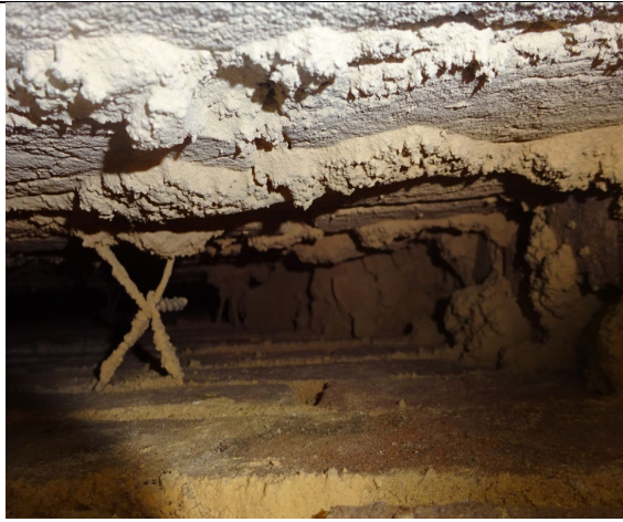
Figure 109: General view to show clear cavity to masonry wall.
