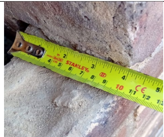
Figure 106: General view to confirm thickness of outer brickwork leaf – 100mm.
