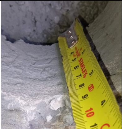
Figure 35: Alternative view to show 20mm pebble dash render and 60mm blockwork outer leaf.
