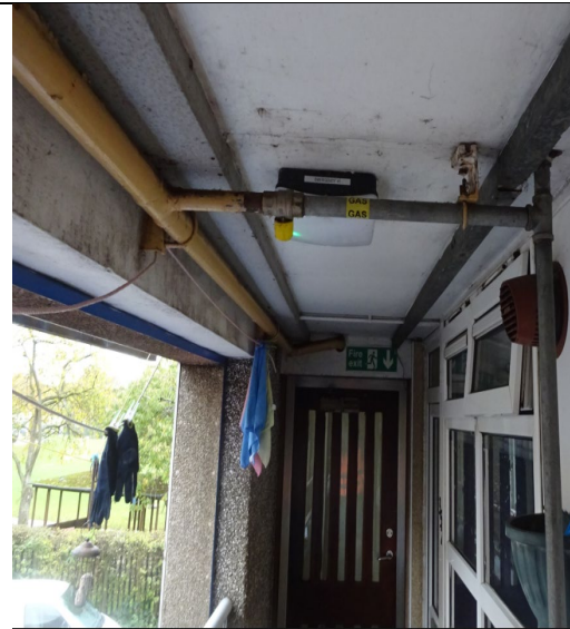
Figure 74: General view to show Fire Door installed at the opposite end of the open access balcony prior to entering the escape staircase and the concrete soffit to the open access balcony.
