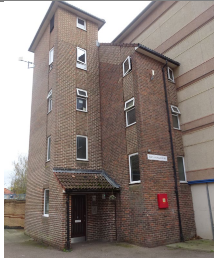
Figure 96: Alternative view of the traditional masonry cavity wall construction to the escape staircase located on the north elevation.
