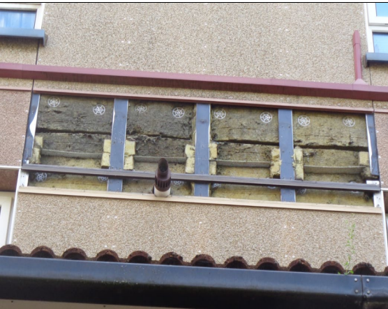
Figure 25: General view to show no horizontal cavity barrier installed at compartment floor location.
