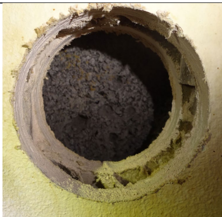
Figure 46: Close up view of the internal Paramount partition lining to the external wall.
