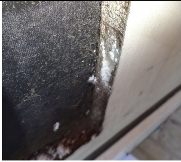
Figure 92: General view to show EPS insulated panel installed at low level to flat entrance door to Flat No. 354 (Harold Court).
