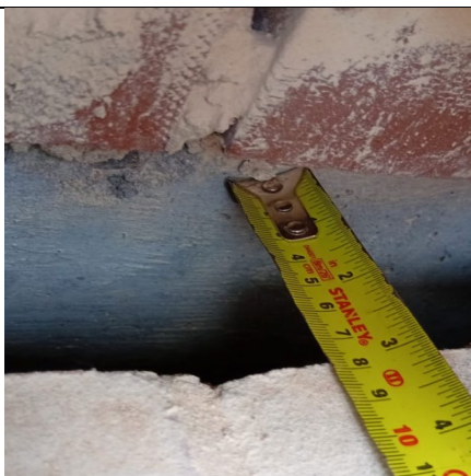
Figure 107: General view to show concrete slab set back from inner leaf to give a clear cavity - 75mm.
