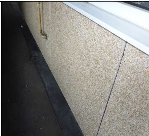
Figure 55: Close up view of the Steni GRP panels installed along the open access balconies.
