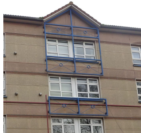
Figure 122: Alternative view of the architectural decorative steel attachments installed to the west elevation.
