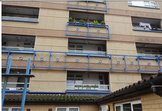
Figure 93: General view to show solid uPVC panels installed at first, second, third and fourth floor levels along the east elevation.
