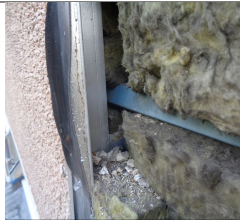
Figure 26: General view to show no vertical cavity barrier installed at compartment wall location.
