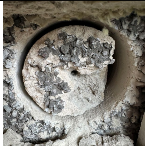
Figure 62: General view to show pebble dash render finish with blockwork inner leaf.
