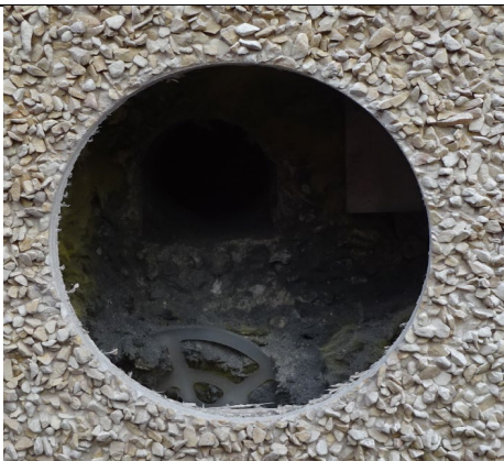
Figure 33: General view to show mineral wool insulation, pebble dash render with blockwork located behind.
