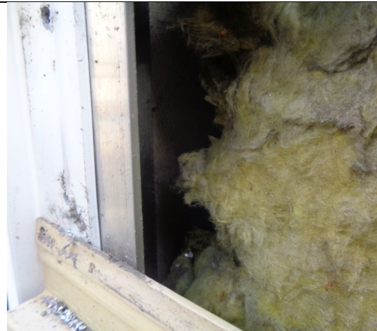
Figure 22: General view to missing insulation to window jamb.
