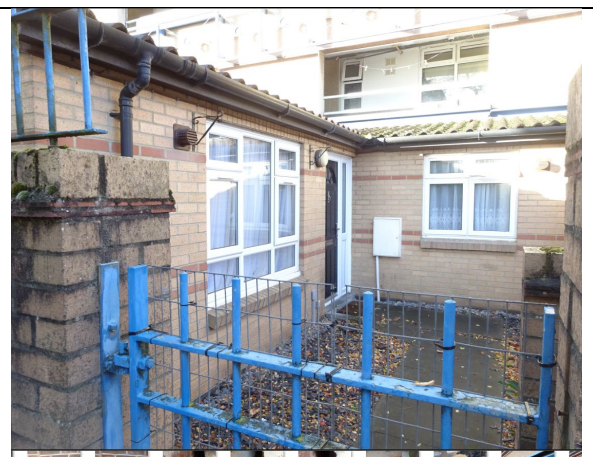
Figure 112: Alternative view of the traditional masonry cavity wall construction to the ground floor flats along the east elevation.
