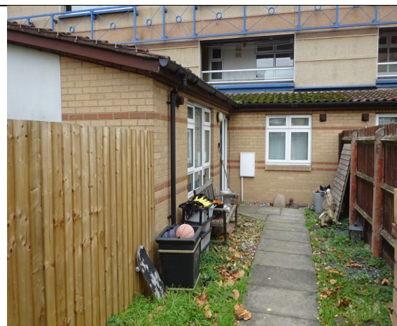
Figure 112: Alternative view of the traditional masonry cavity wall construction to the ground floor flats along the east elevation.
