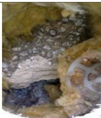
Figure 33: General view to show mineral wool insulation, pebble dash render with blockwork located behind.
