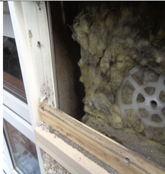
Figure 22: General view to missing insulation to window jamb.
