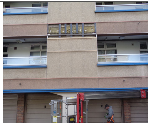
Figure 76: General view of compartment floor location to show no horizontal cavity barrier at compartment (Taken from Queens Court 2021).
