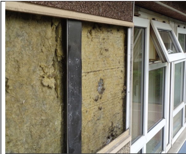
Figure 29: Close up view to show Steni GRP panels and mineral wool insulation.
