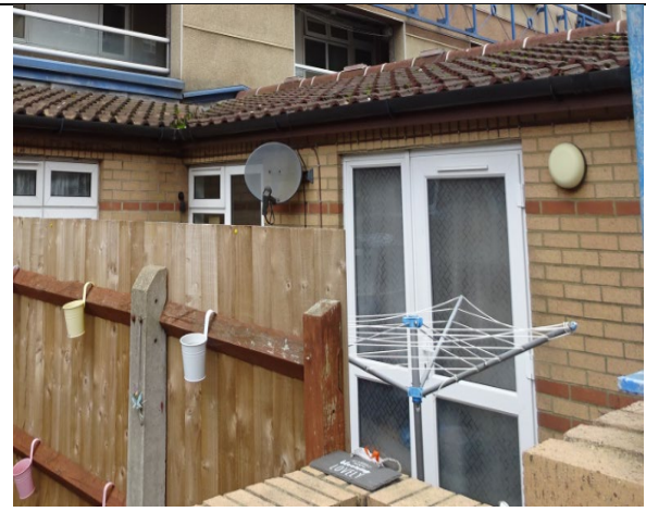
Figure 114: Alternative view of the traditional masonry cavity wall construction to the ground floor flats along the east elevation.
