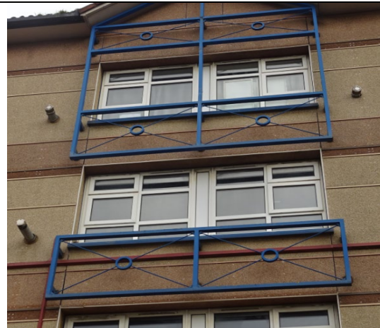
Figure 122: Alternative view of the architectural decorative steel attachments installed to the west elevation.
