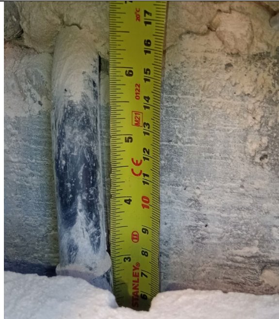
Figure 110: General view to confirm concrete slab thickness to escape staircases – 160mm.
