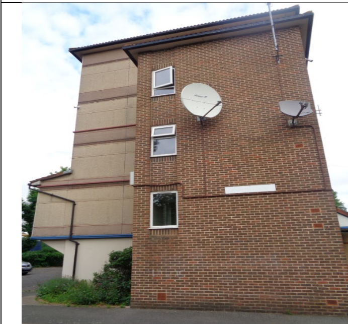
Figure 3: Rear (South) elevation of the building.
