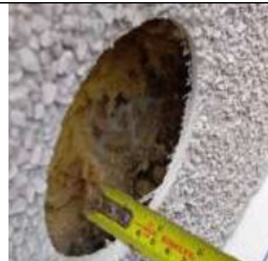
Figure 32: General view to show Steni GRP rainscreen cladding panel, cavity void and mineral wool insulation.
