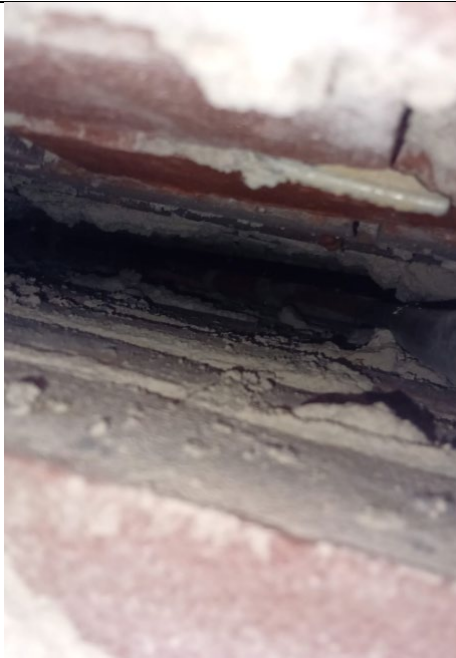
Figure 109: General view to show clear cavity to masonry wall.
