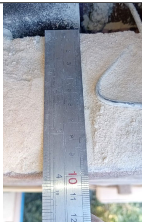
Figure 107: General view to confirm thickness of outer brickwork leaf – 100mm.
