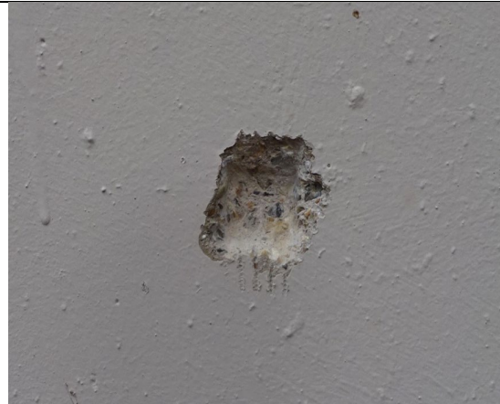
Figure 116: Close up view of the sample location to confirm solid concrete shear wall.
