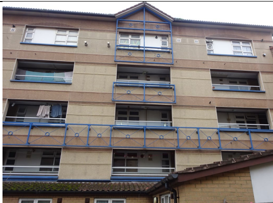
Figure 93: General view to show solid uPVC panels installed at fourth floor level along the east elevation.
