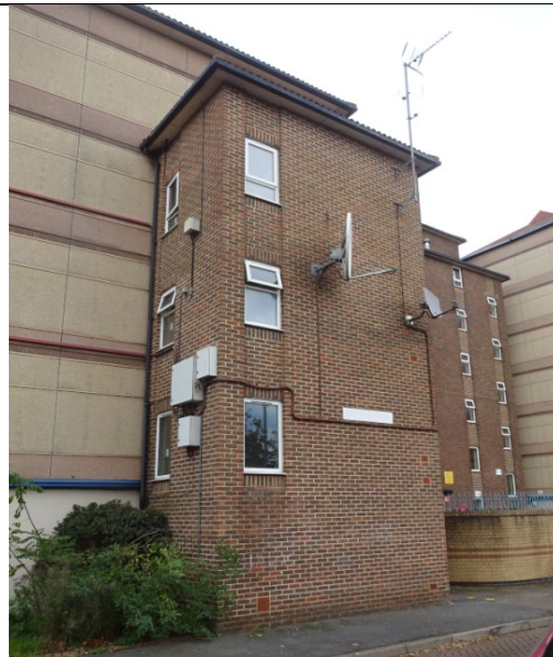
Figure 98: General view of the traditional masonry cavity wall construction to the escape staircase located on the south elevation.
