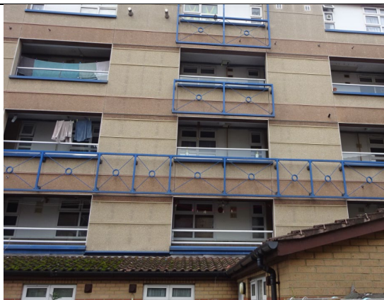
Figure 75: General view of External Wall Type #4
