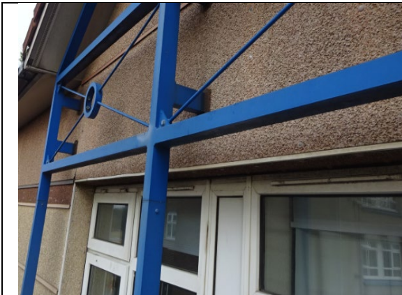
Figure 125: Close up view of the decorative architectural steel attachments installed (Taken from Alexandra Court).
