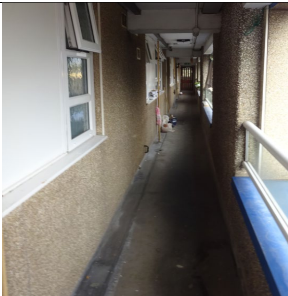
Figure 53: General view of the Steni GRP panels installed along the open access balconies along the east elevation at first floor level.
