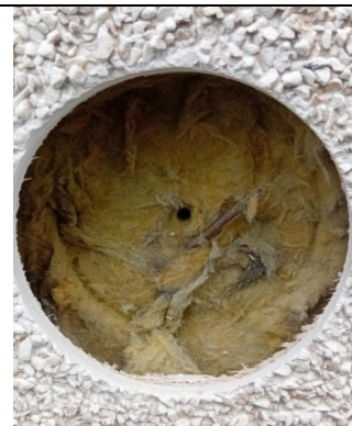
Figure 40: Close up view to show Steni GRP rainscreen cladding panel, cavity void and mineral wool insulation.
