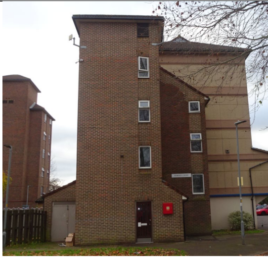
Figure 95: General view of the traditional masonry cavity wall construction to the escape staircase located on the north elevation.
