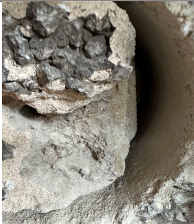
Figure 63: Alternative view to show pebble dash render finish with blockwork inner leaf.
