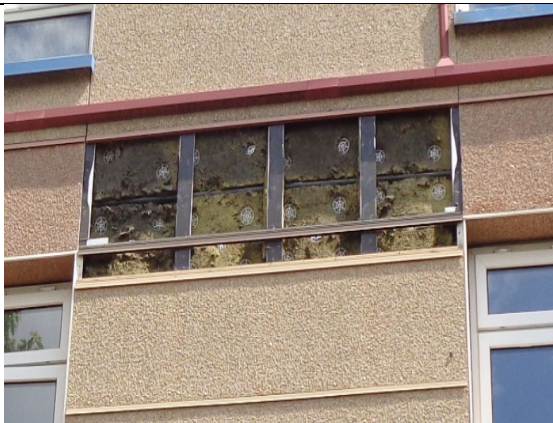
Figure 25: General view to show no horizontal cavity barrier installed at compartment floor location.
