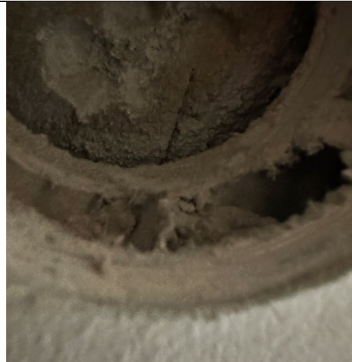
Figure 68: Close up view of the internal Paramount partition lining to the external wall.
