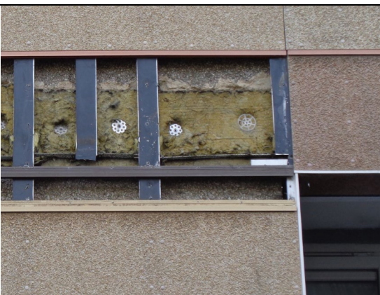
Figure 77: Close up view of compartment floor detail, which shows mineral wool insulation installed at compartment floor location, but this does not fully fill the void behind the Steni GRP rainscreen cladding panel (Taken from Queens Court 2021).
