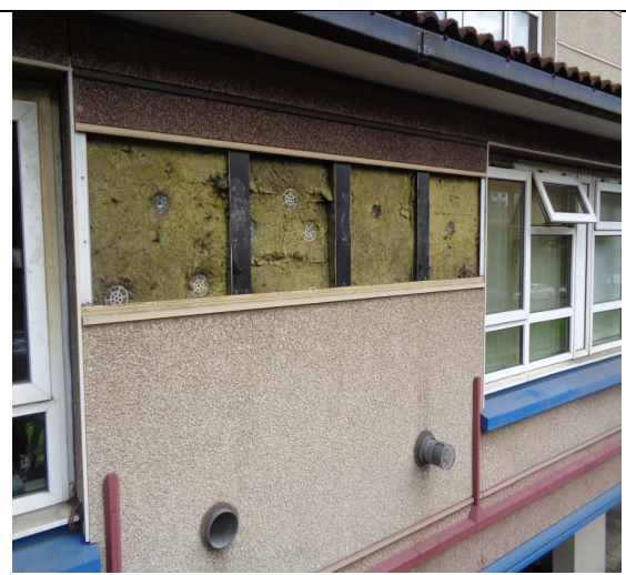
Figure 28: Alternative view of External Wall Type #2.
