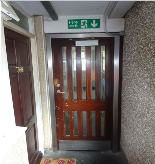
Figure 73: General view of Fire Door installed at the end of the open access balcony prior to entering the escape staircase.
