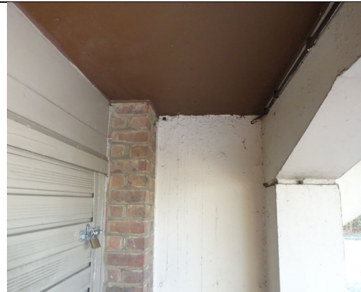
Figure 118: Close up view to show reinforced concrete wall and frame to the west elevation.
