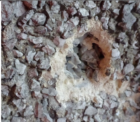
Figure 85: Close up view to show pebble dash render finish installed over Wimpey no fines concrete.
