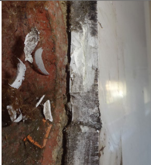
Figure 91: Close up view to show 20mm solid uPVC panel.
