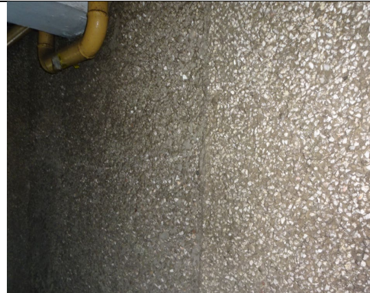
Figure 86: General view of pebble dash render finish to external wall of first floor open access balcony along the east elevation.
