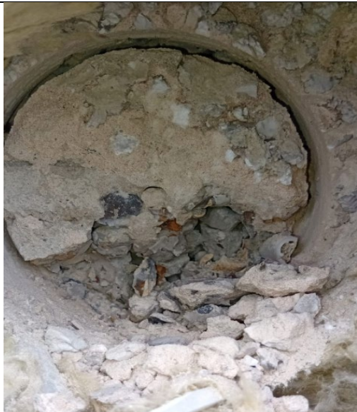
Figure 21: Close up view to show pebble dash render with Wimpey no fines concrete located behind render finish.
