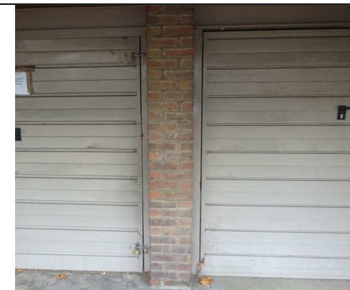
Figure 120: General view to show solid masonry wall located between garages.
