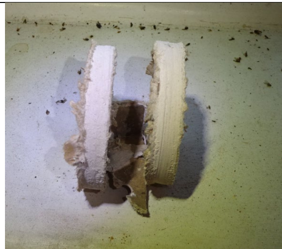
Figure 70: Close up view of Paramount partition lining board which comprises of two layers of 10mm plasterboard with an 18mm honeycomb cardboard core.
