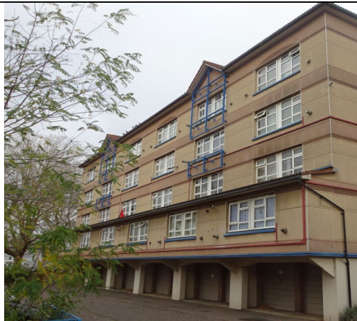
Figure 121: General view of the decorative architectural steel attachments installed to the west elevation.
