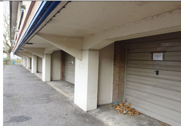
Figure 117: General view of the reinforced concrete frame and concrete floor to the west elevation. NB. that the garages are recessed back from the main elevation.
