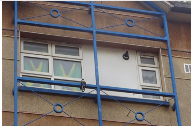
Figure 94: Close up view of the solid uPVC panels installed at fourth floor level along the east elevation.
