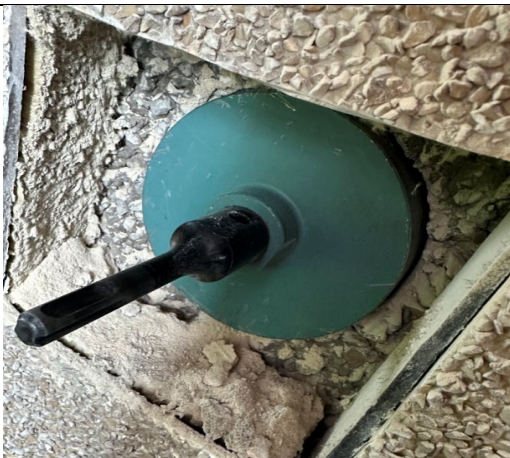
Figure 65: General view to show core hole drill bit at maximum depth drilling into blockwork inner leaf.
