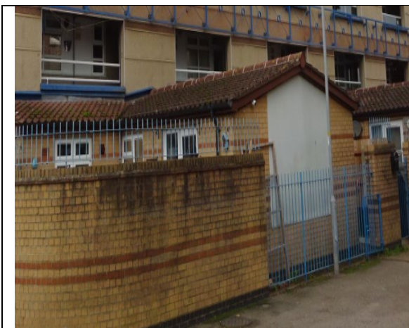
Figure 111: General view of the traditional masonry cavity wall construction to the ground floor flats along the east elevation.
