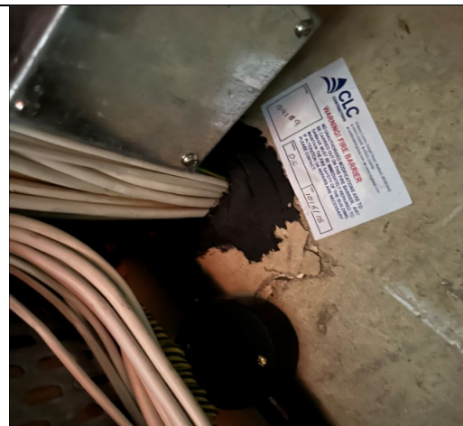
Figure 102: General view to show fire stopping works including ID labels completed to riser cupboards located in escape staircases.
