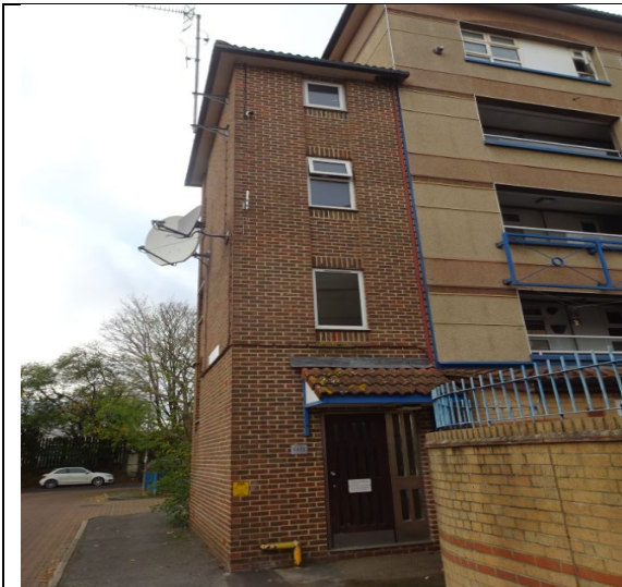
Figure 99: Alternative view of the traditional masonry cavity wall construction to the escape staircase located on the south elevation.
