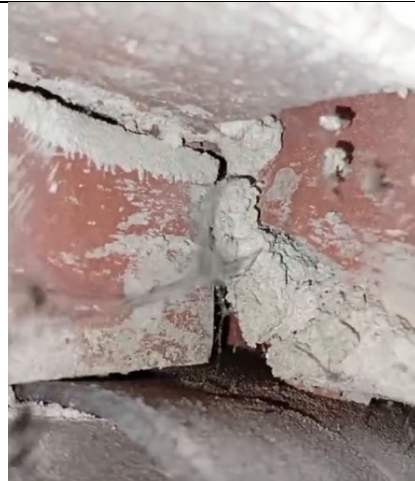
Figure 106: Alternative view to show masonry brickwork closing the cavity.
