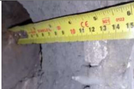
Figure 35: Alternative view to show 20mm pebble dash render, 60mm blockwork outer leaf and 50mm clear cavity.
