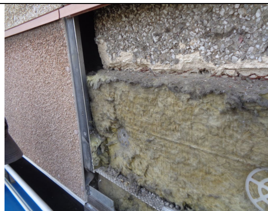
Figure 78: Alternative view of compartment floor detail, which shows mineral wool insulation installed at compartment floor location, but this does not fully fill the void behind the Steni GRP rainscreen cladding panel and the concrete floor slab (Taken from Queens Court 2021).
