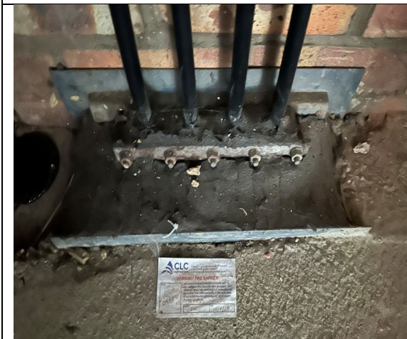
Figure 101: General view to show fire stopping works including ID labels completed to riser cupboards located in escape staircases.
