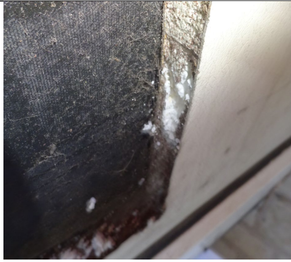
Figure 92: General view to show EPS insulated panel installed at low level to flat entrance door to Flat No. 354.
