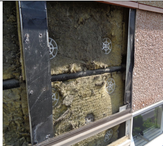
Figure 16: Close up view to show mineral wool insulation.
