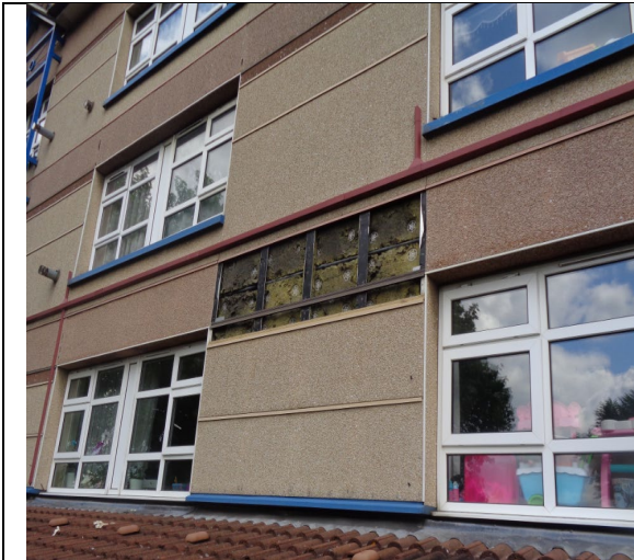
Figure 15: General view of External Wall Type #1.
