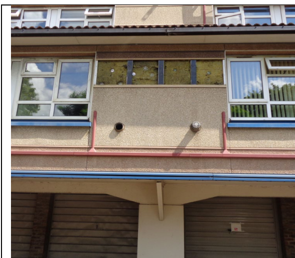
Figure 27: General view of External Wall Type #2.
