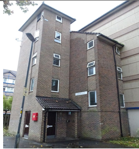
Figure 96: Alternative view of the traditional masonry cavity wall construction to the escape staircase located on the north elevation.
