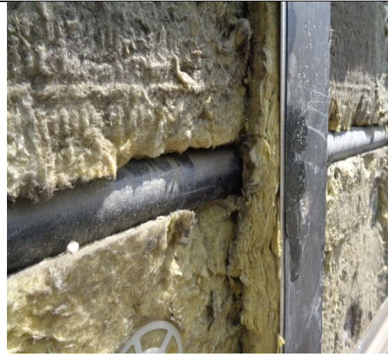
Figure 24: General view to show service pipes / cables located with mineral wool insulation.
